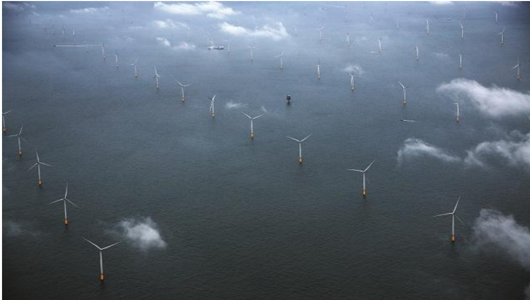
London Array, United Kingdom (630 MW)
