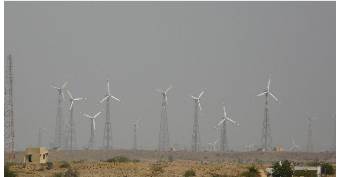
Jaisalmer wind park, Rajasthan (1064 MW)
